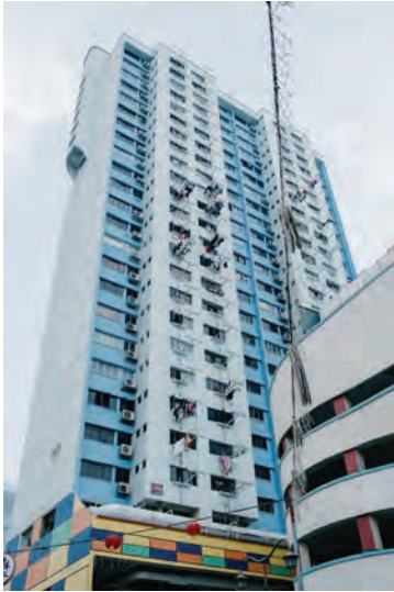
Public housing high-rise in Chinatown
